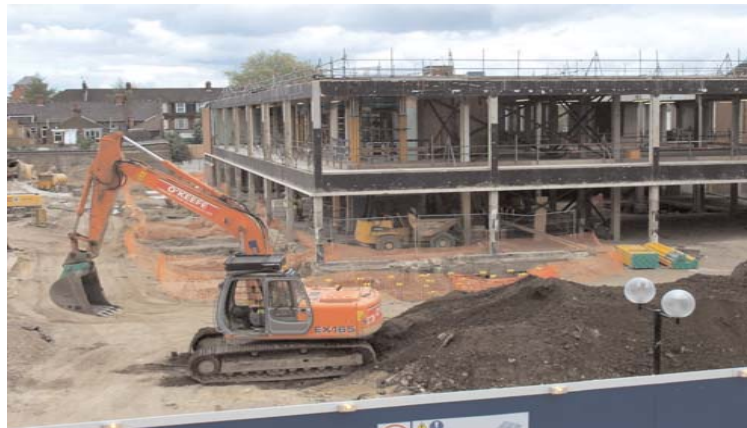
Construction of the Lifelong Learning Centre (March 2005)
