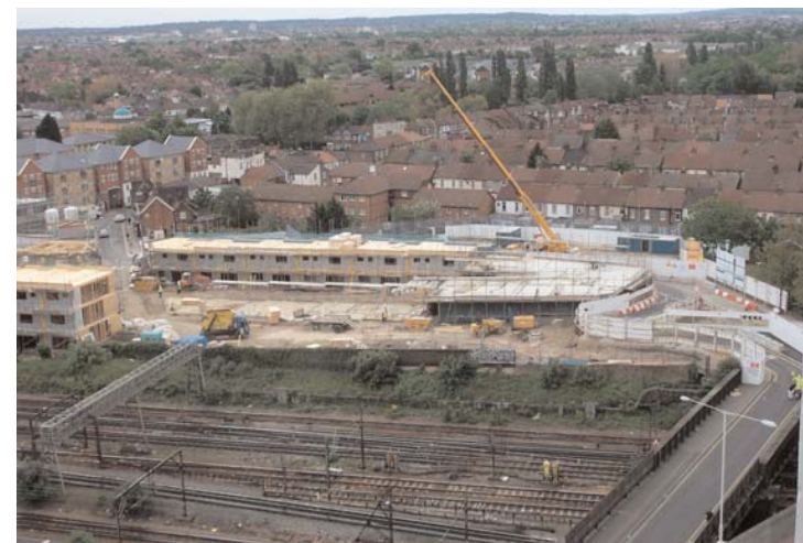
Construction at Tanner Street Gateway
